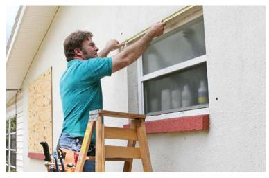
Hurricane research studies have shown that on average; homes built under the 2002 Florida Building Code sustained less damage and when paired with shutters may be safe to stay in as long as they are not in an evacuation area. Homes built between 1994 and 2001 under the Standard Building Code sustained more damage and homes built before 1994 fared even worse. Before storm season begins, take the following steps to protect your home:
